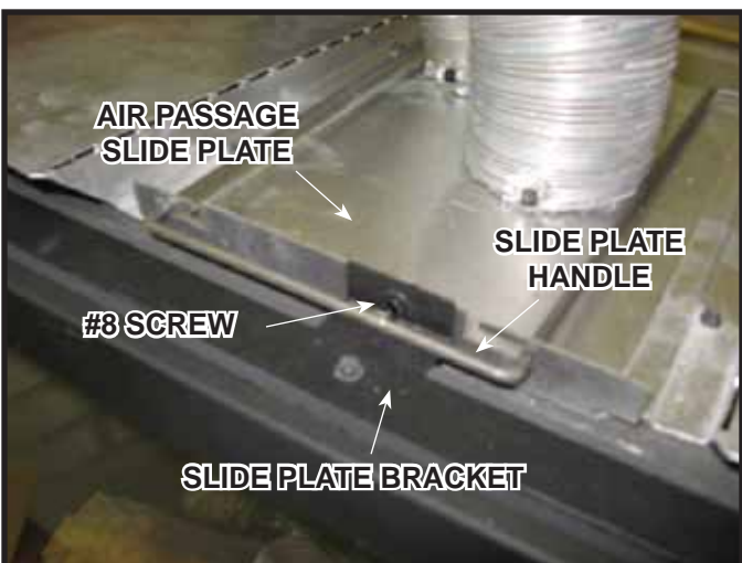
Figure 8.3 Slide Plate Components
